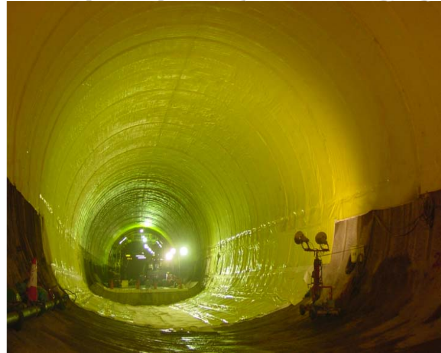
High Endurance Tunnel-Arch Structure Method
