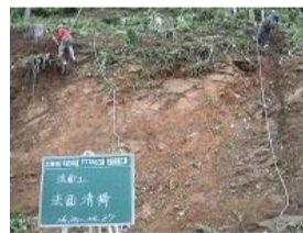
①法面清掃
