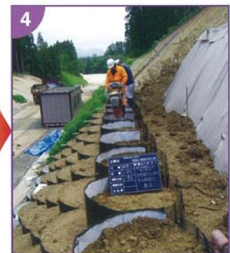
[中詰材・裏込材転圧]
