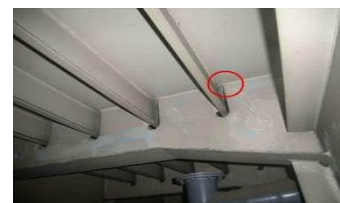
鋼床版のき裂
